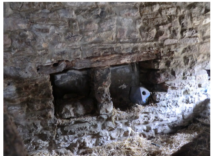
Double shelves / lantern holes and wooden lintel
